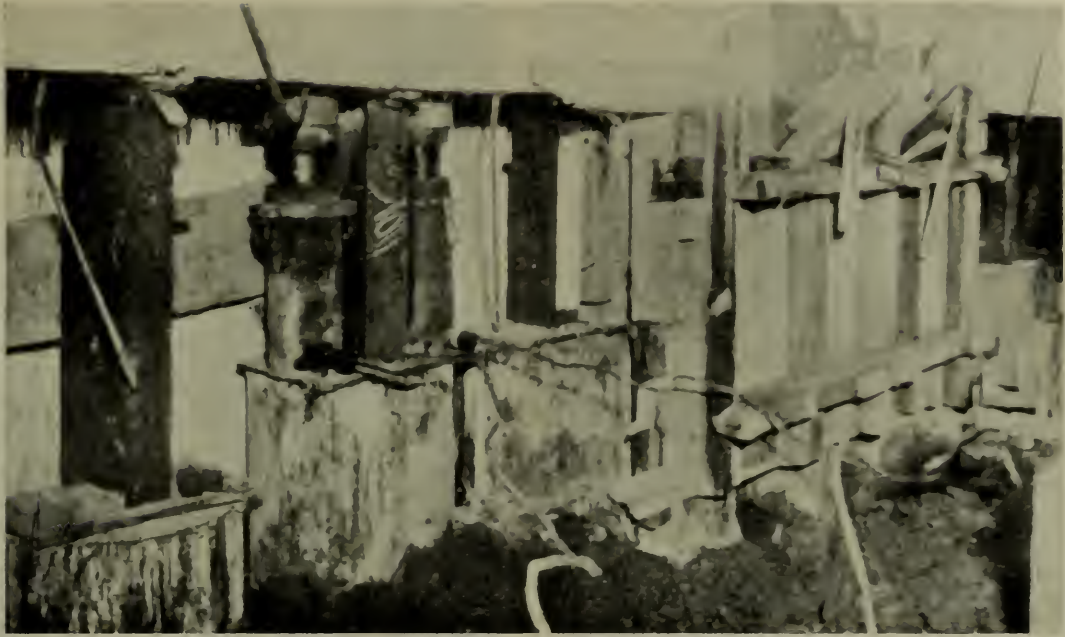
FIG. 3. TESTING "PRETEST" PILES UNDER EXTERIOR WALLS.
